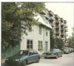
Three phases of straw bale in the city! This straw bale residence in Montreal was granted full approval under the city's strict building codes.
